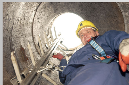
Confined space access
