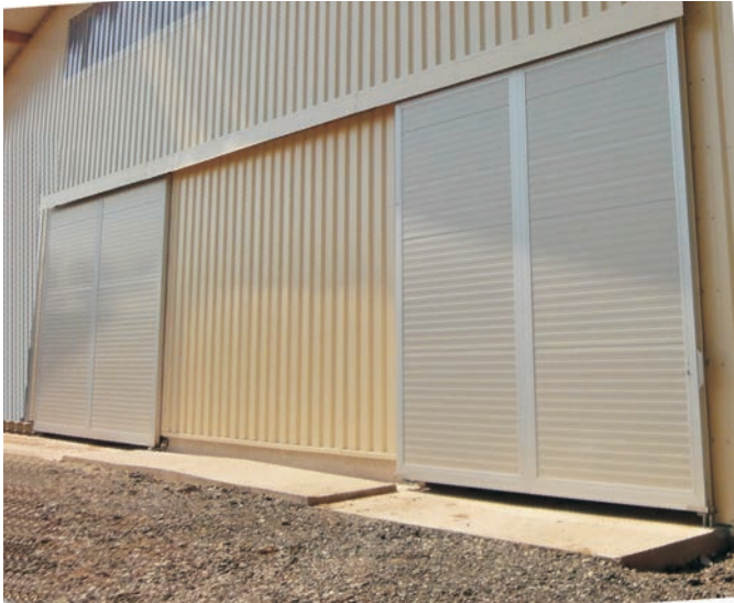
Sliding door, aluminum frame system with ISO panels, folding plates and hook lock.
