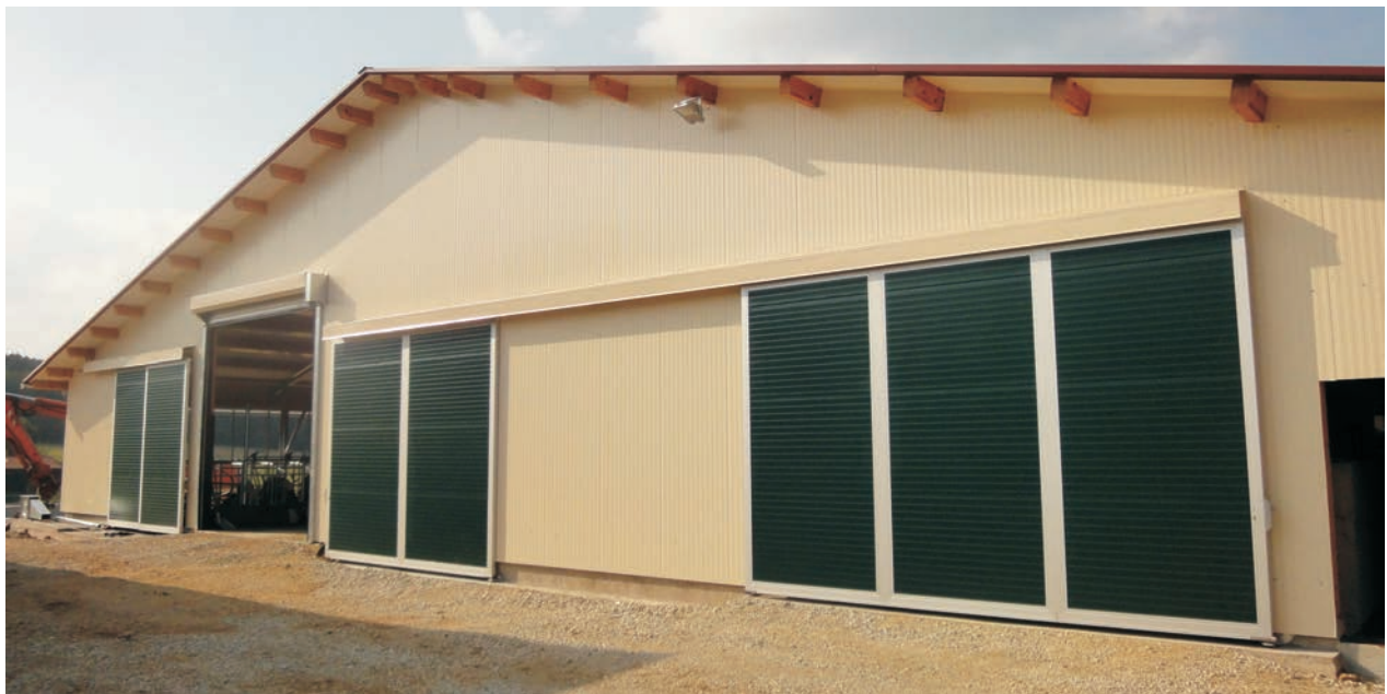
Sliding door, aluminum frame system with ISO panels, floor guidance guide track on the door leaf.
