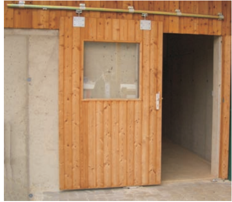
Sliding door with viewing window, wall brackets, folding plates and hook lock.
