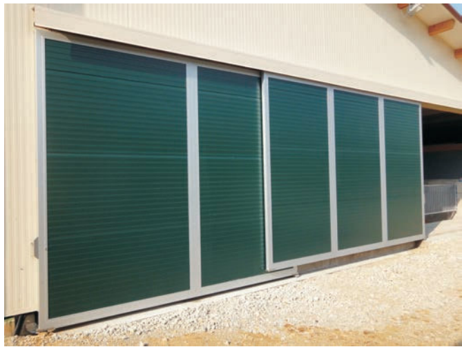
Sliding door, aluminum frame system with ISO panels, folding plates and hook lock.
