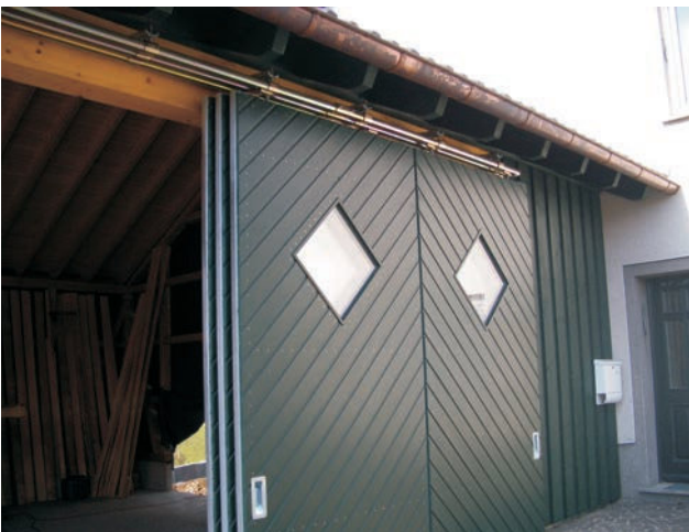
Modular door design with double wheel hangers and integrated door. Floor guidance with guide track on the door leaf.
