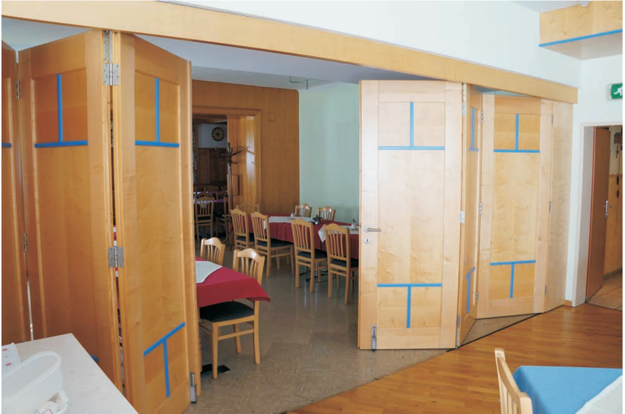
Folding door with three leaves on each side and floor recessed guide track. Ceiling support brackets and top corner bracket Type C. Double wheel hangers and pedestrian door.
