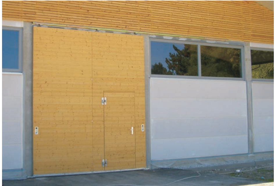
Modular door design with double wheel hangers and integrated door. Floor guidance with guide track on the door leaf.
