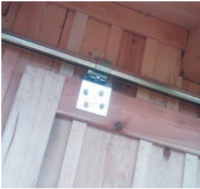
Folding plate on the door panel with suspension bracket
