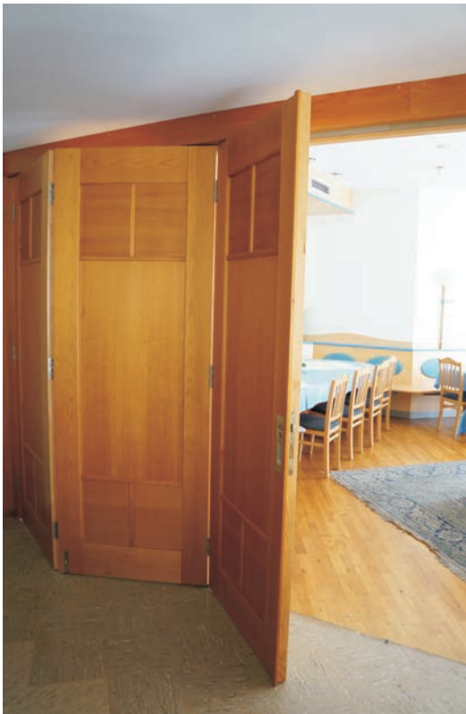
Recessed guide track eliminates the trim hazard across the threshold. Doors with flush handles.
