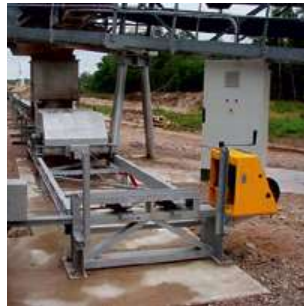
△ Conveyor belt tensioning.
