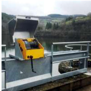
△ Opening of a sluice gate.
