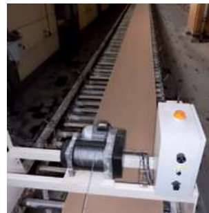
▶ Moving a trolley on a conveyor during maintenance operation.
